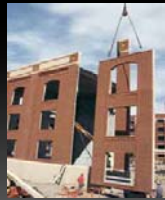
Panel Erection
