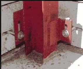
4-Way Adjustment Connection at Column
